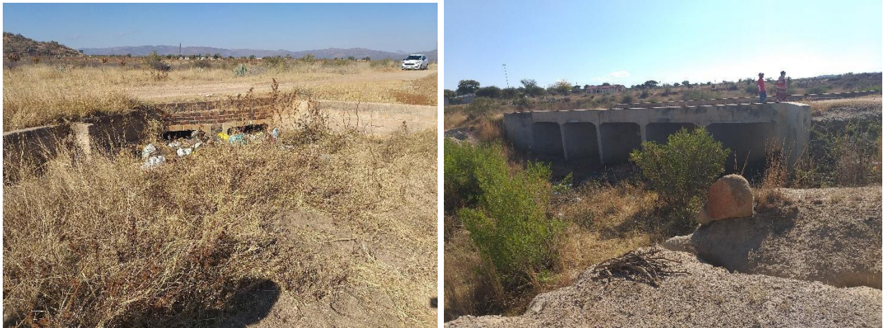
Figure 288-2: Existing culvert structures
